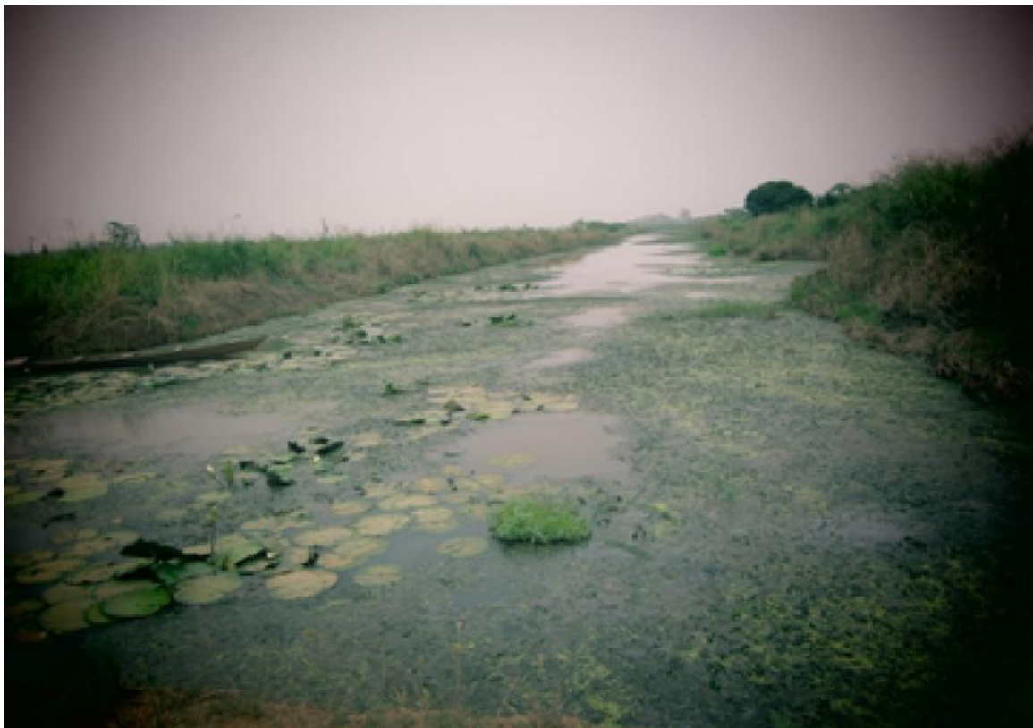
Figure 10: An Irrigation Canal which also serves as an alternative water source
