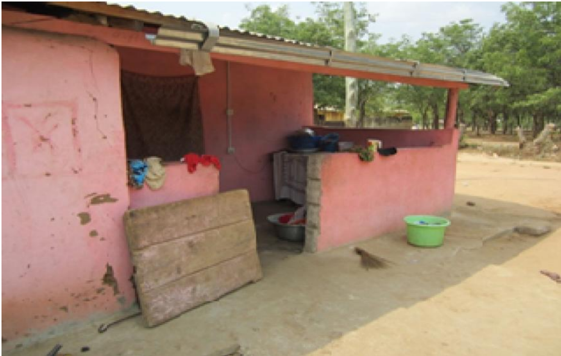
Figure 9: An example of a cement house in Lanor (a pipe community)
