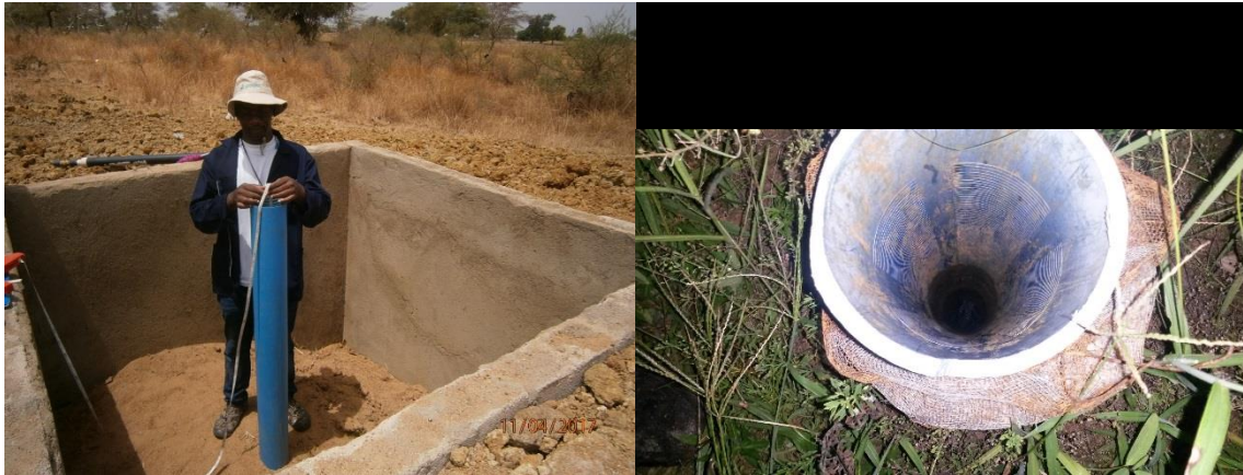
Figure 3-4. Infiltration bed showing constructed blockwork and screen with mesh
