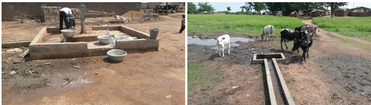
Figure 5-1. Poor sanitation around community borehole
