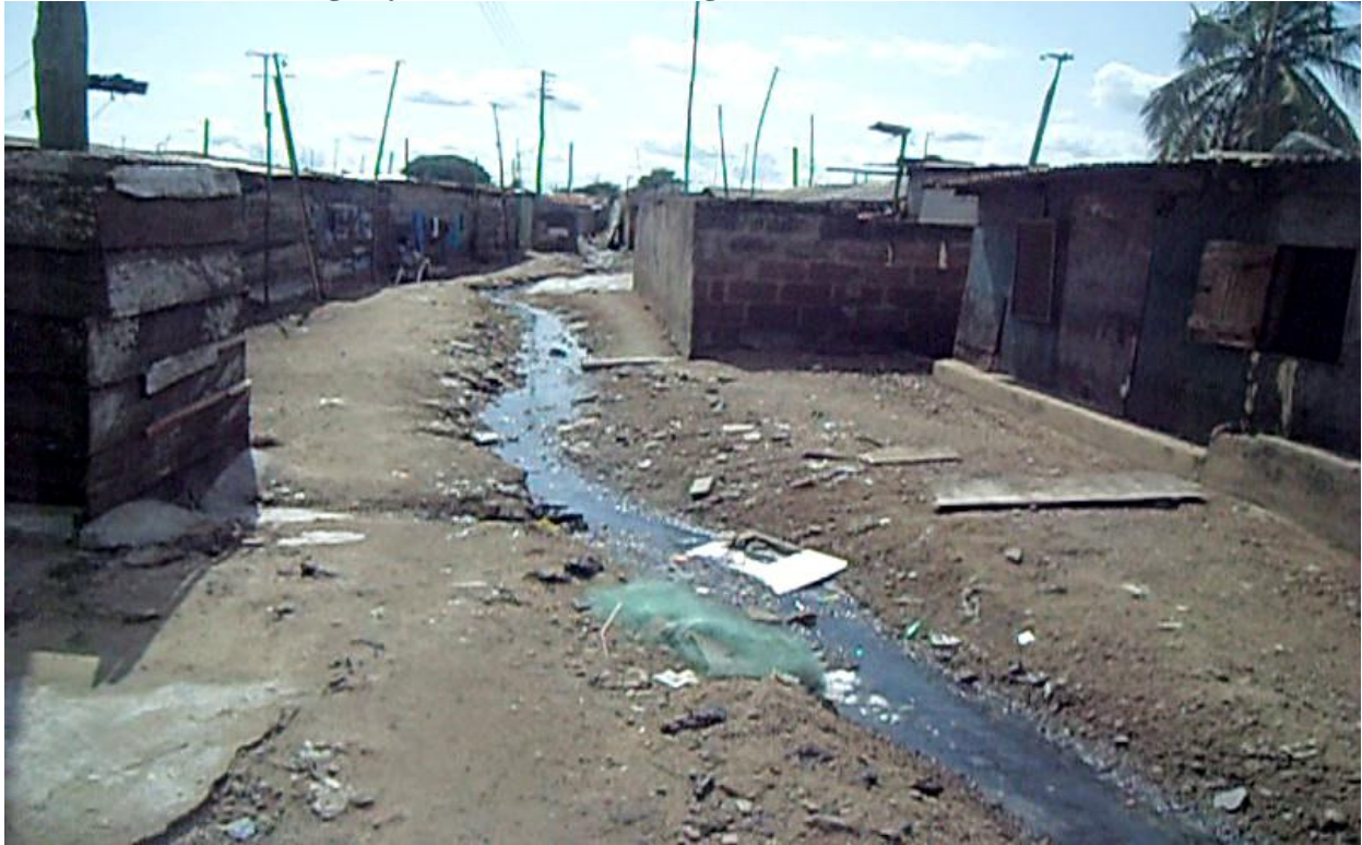
Plate 3.3 Poor Drainage System within Dwellings
