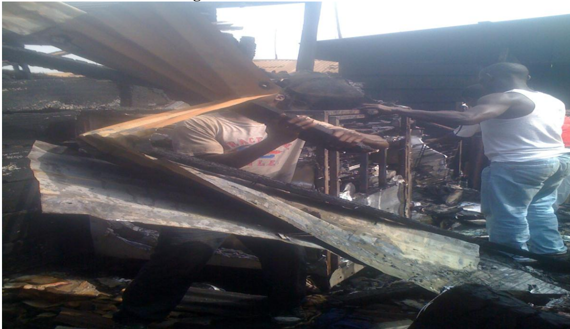
Plate 5.1 Residents Knocking down Structures to Create Fire Breaks
