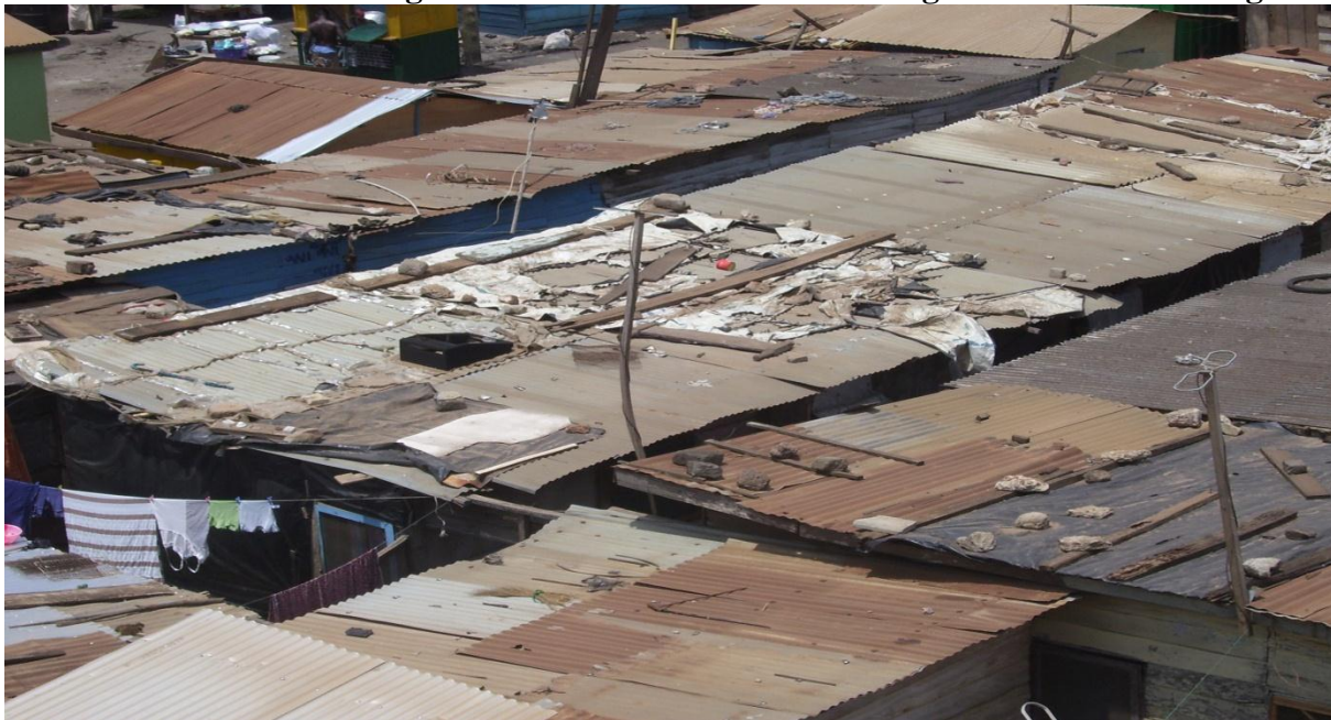
Plate 4.3 The Use of Corrugated Aluminium Sheets in Roofing of Informal Dwellings
