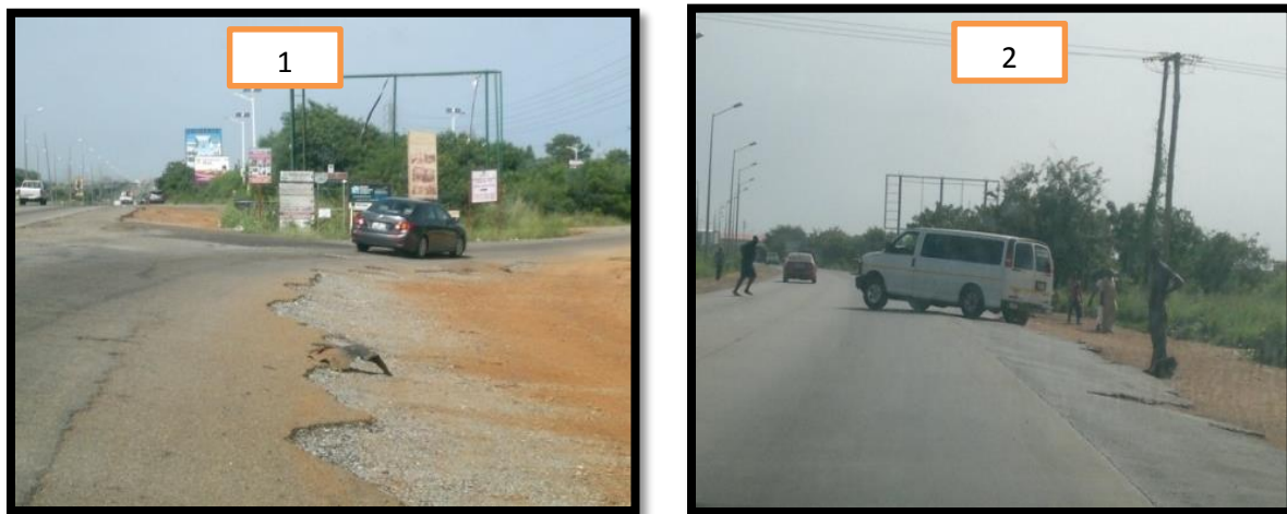
Figure 4.9: Sections of Accra-Tema Motorway Showing Illegal Entries and Exits
