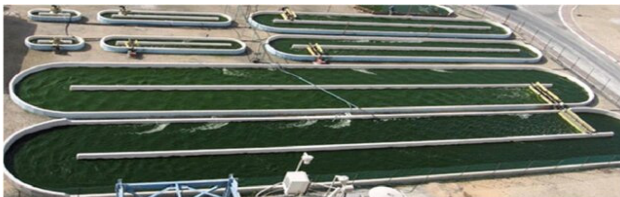
Figure 2. Raceway pond system with moving paddles [82].
