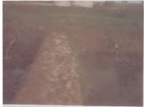
Plate 3.15 Pond filling (Inlet pipes at work)
