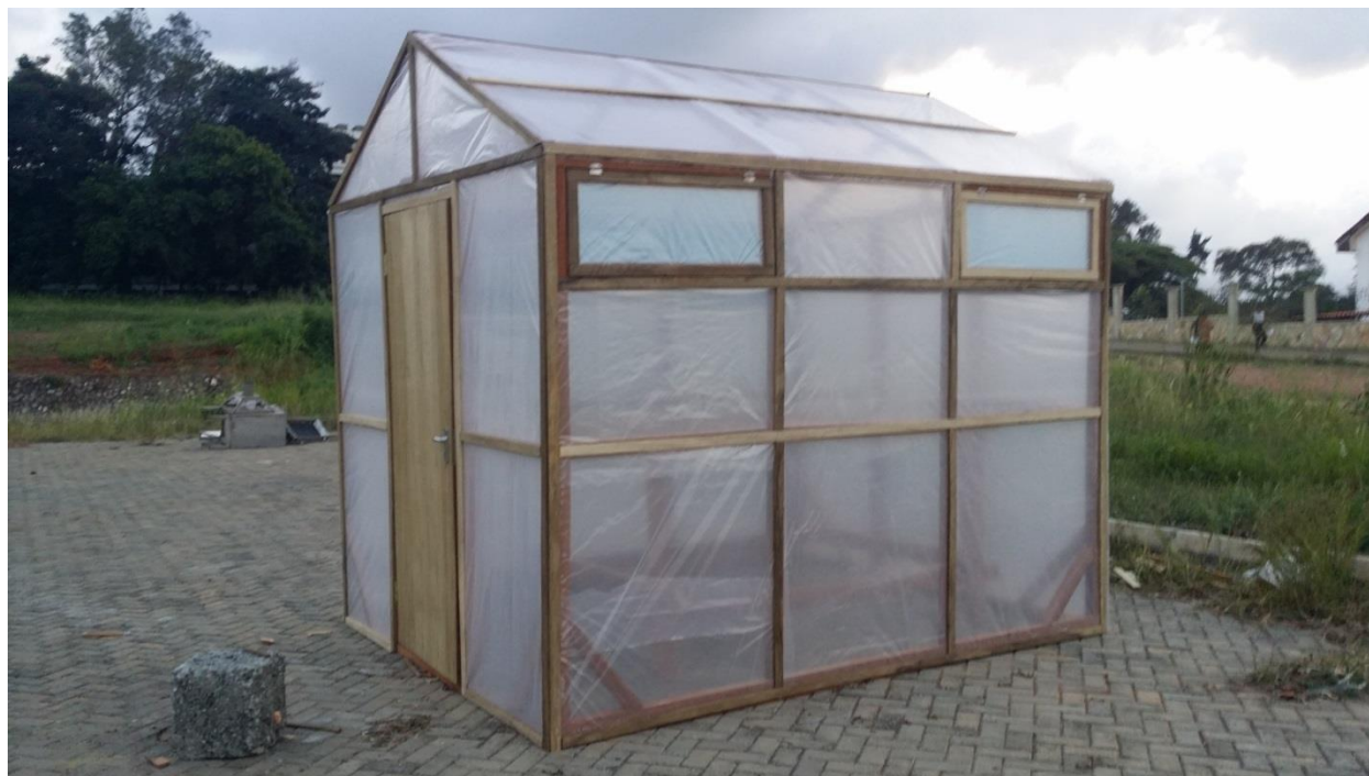
Illustration 1. The Greenhouse type solar dryer
