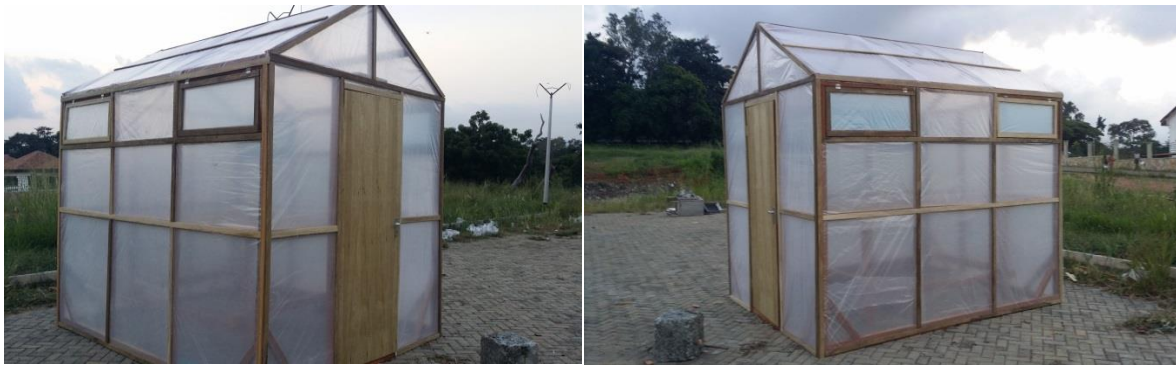
Illustration 8. Completed GTSD with polyethylene cover
