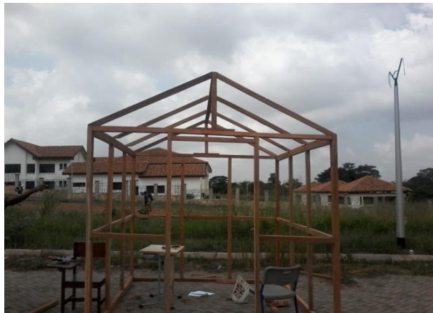
Illustration 6. Base and roof framework of GTSD
