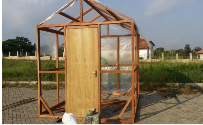
Illustration 7. Completed framework with door of GTSD
