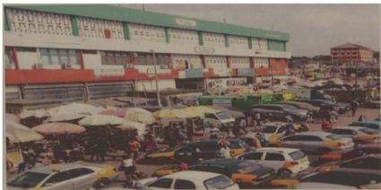
Figure 3: Kaneshie market showing the complex building with various activities outside the building
