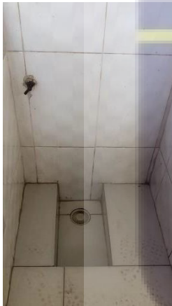
Plate 4. Examples of floor mounted indoor urinal (A). B is a wall mounted pot in an indoor urinal.
