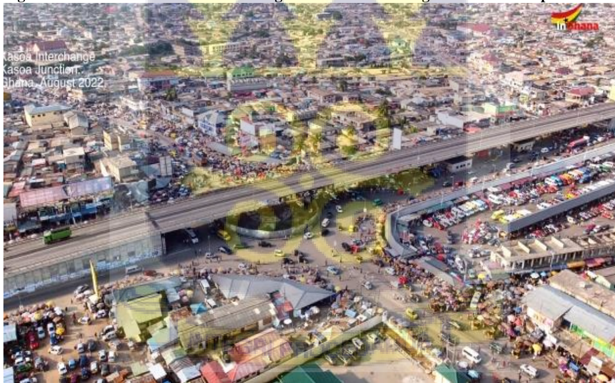
Figure 4.4: Aerial view of ASEM showing the Kasoa interchange and its urban sprawl
