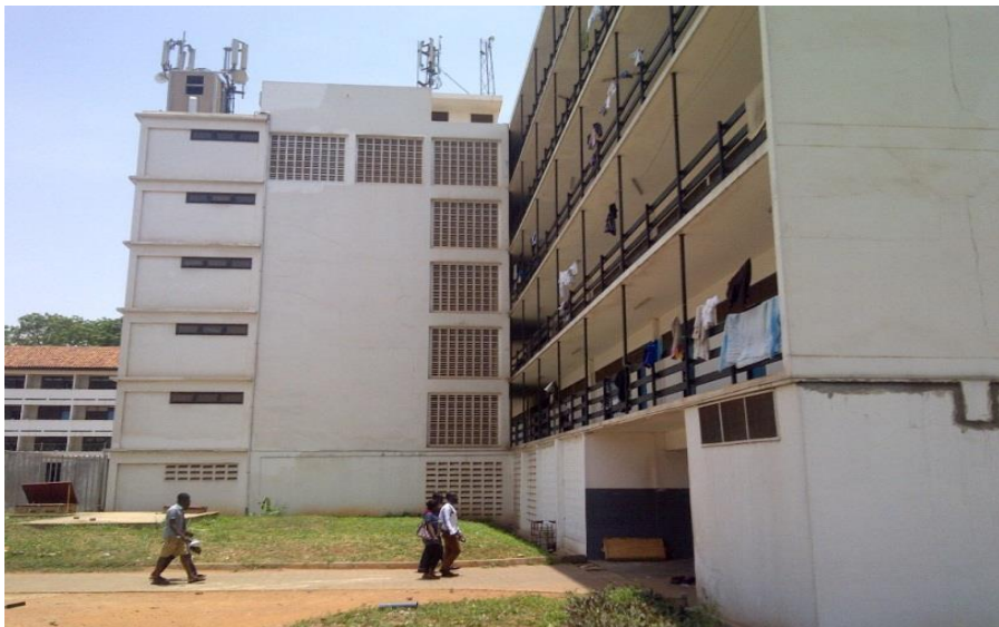
Plate 3.3: Site for rooftop base station eleven (11)
