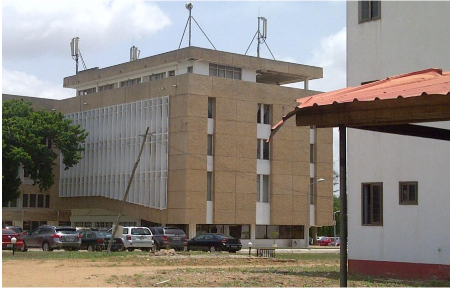
Plate 3.2: Site for rooftop base station twelve (12)
