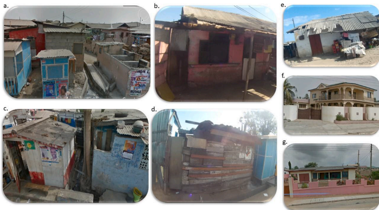
Fig. 3. Different structures digitized from the SVs. Included informal wooden structures referred to locally as “kiosks”, houses with scavenged roofing, bathrooms connected to open drains and well-designed houses with good roofing and painting. D is an example of a structure ranked as 1 whilst F is ranked as 5.
