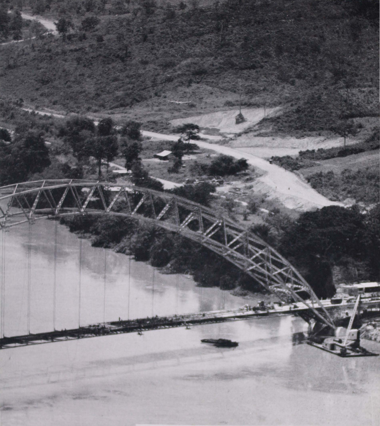
The great bridge over the River Volta at Adomi, one of the biggest in Africa, was completed in 1956. It links two parts of the country which had hitherto only been accessible to each other by ferry. And it is a key piece in the construction of the new eastern highway which runs from Accra to Bawku
