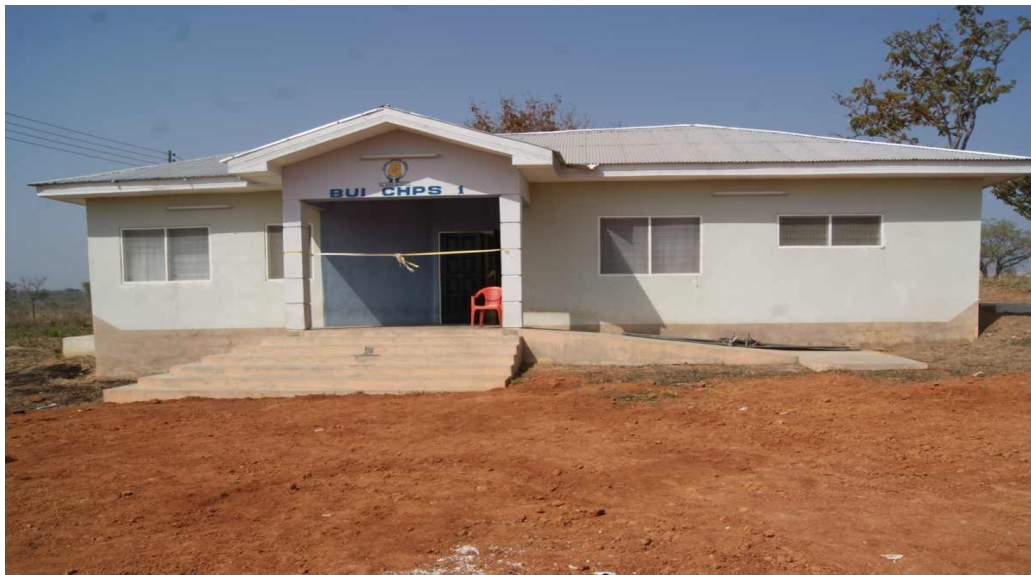
Figure 4.2 CHP compound for health delivery
