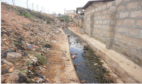
Peripheral drains to carry leachates from decommissioned landfill site at Mallam
