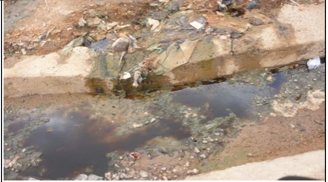
Peripheral drains to carry leachates from decommissioned landfill site at Mallam
