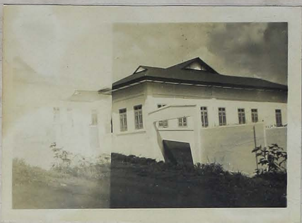
A MODERN BUILDING.
