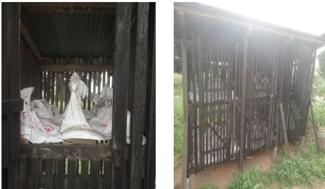
Plate 3.1 Constructed Ventilated Crib at University of Ghana Farm
