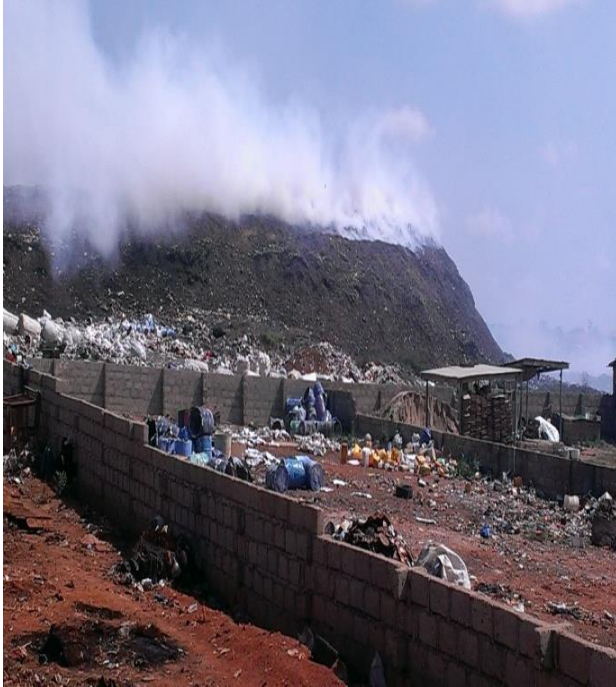
Plate 3: State of the dump site
