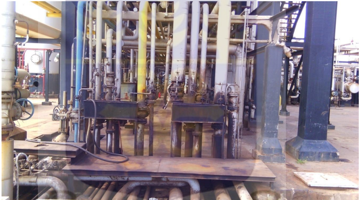
Figure 3.1 Sampling point of finished product from the CDU and RFCC of TOR.
