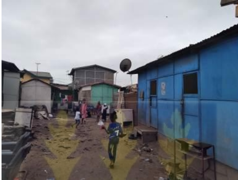
Figure 6.1: Typical wooden (Plywood) Structures at Old Fadama
