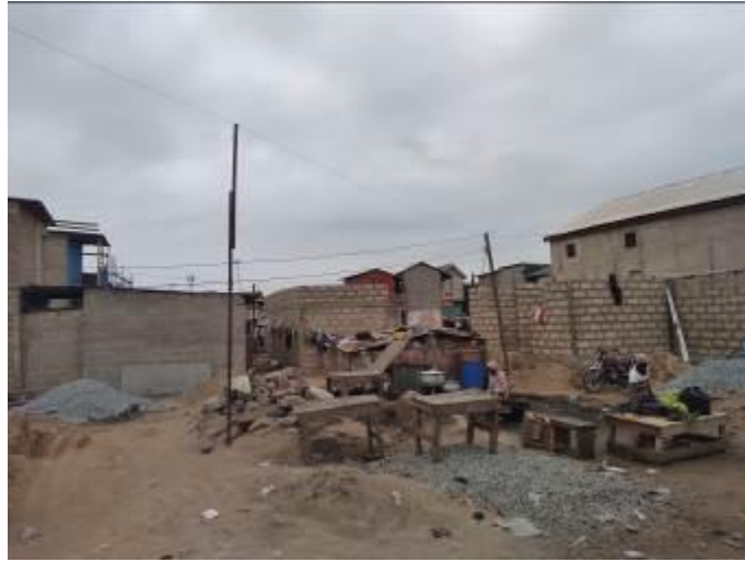
Figure 4.2: New Block Construction ongoing in Old Fadama
