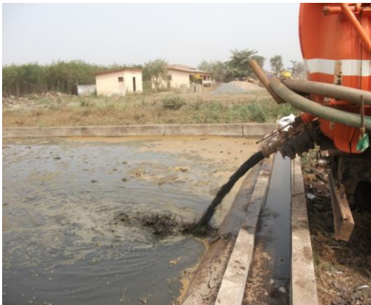
Plate 3.2: A cesspit emptier dislodging onto the drying bed.
