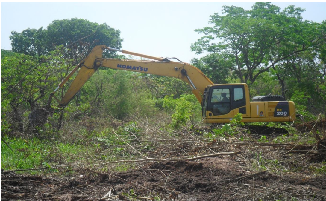
Figure 6: The Komatsu PC 200 Tractor de-stumping the field off trees and shrubs
