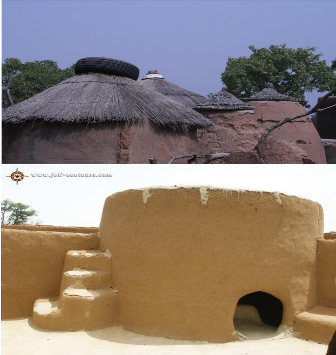
Figure 4.9: A Mud and Thatch/Grass Roof and Mud with Soil Roof House at Paga
