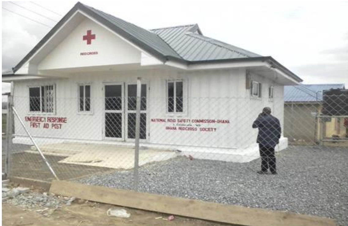
Figure 3. 3: Emergency Rapid Response Post constructed by NRSC
