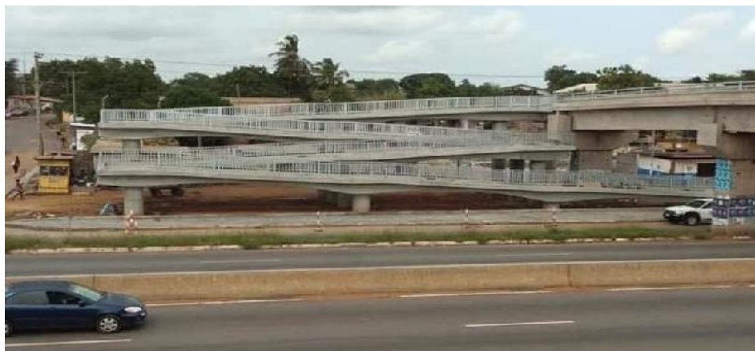
Figure 3. 4: Madina- Adenta overhead bridge
