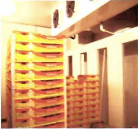
Appendix 12: Holding Room
