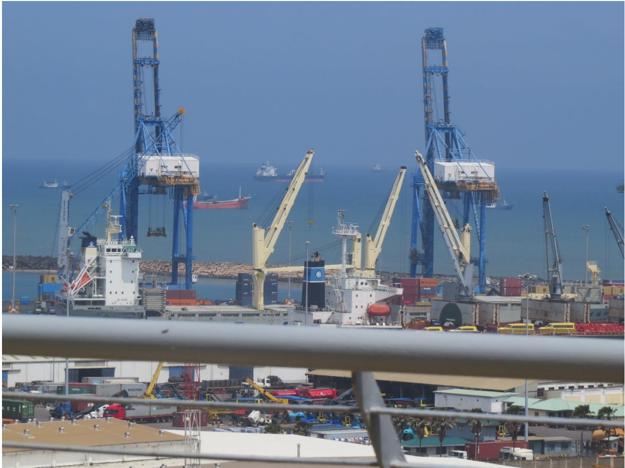
Figure 19: Newly Acquired Mobile Harbour Cranes for Tema Port
