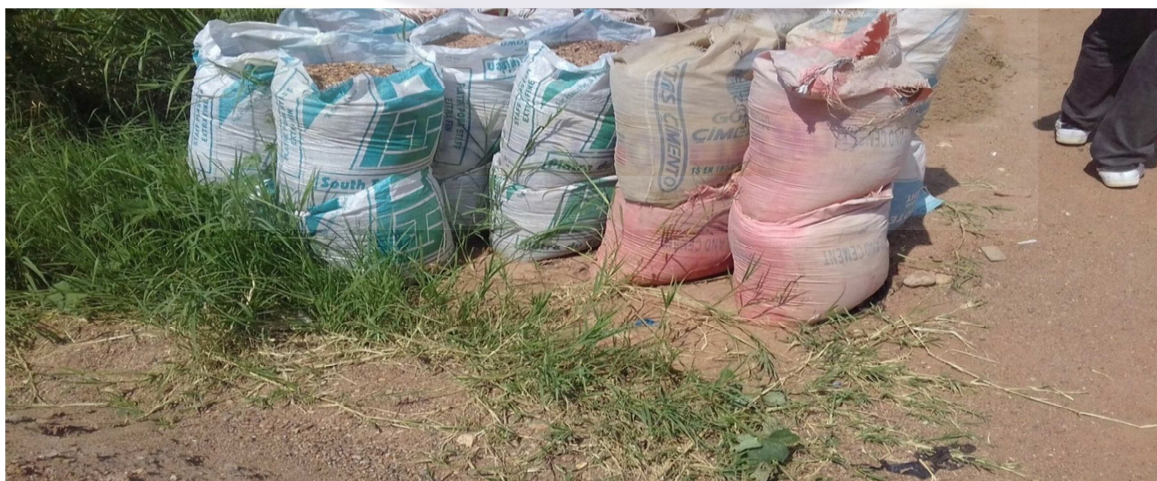
Plate 4.6: Sand Bags field to Block flood water at Tse-Addo
