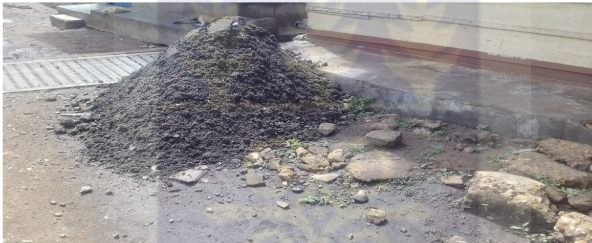
Plate 4.5: Sand Cleared from a Choked Gutter in Front of a Building in Kenan Factory
