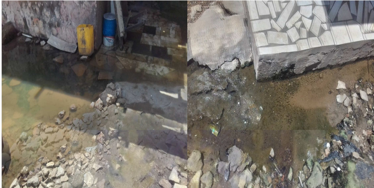
Plate 4.1: Forcourts of some Buildings in Pentecost Down
