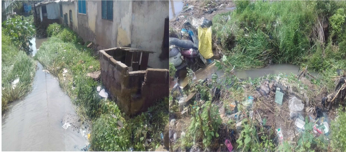
Plate 4.2: Pictures showing the Main Drain at Kenan Factory
