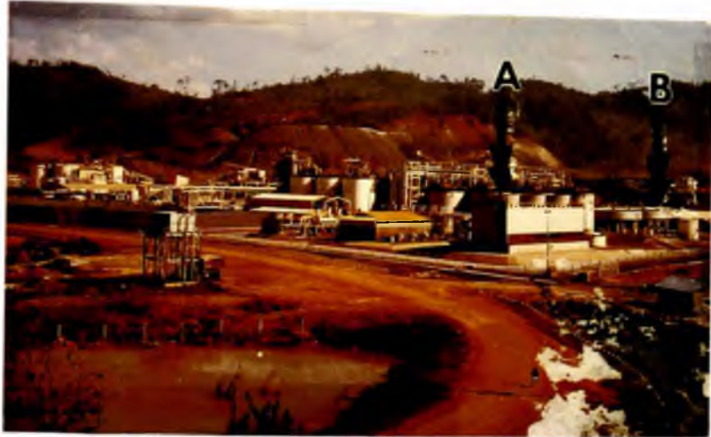
Figure 1 Photograph showing the sulphide treatment plant (STP) at Obuasi. A= reactor tank, B= settling tank.
