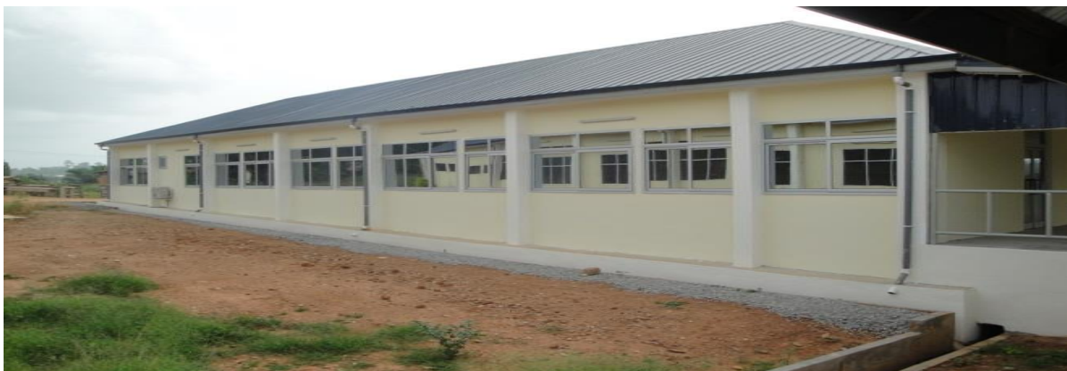
iv. Figure 4.4 New Operating Theatre for the New Abirem Govt. Hospital
