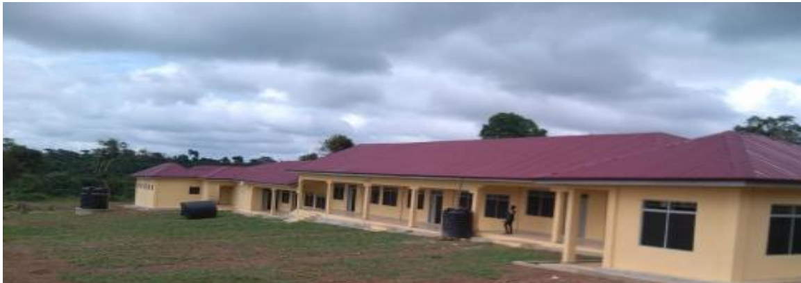
ii. Figure 4.1 girls vocational dormitory constructed by the NGRL at Afosu
