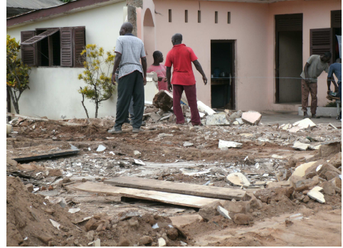
Fig. 5. Some citizens witnessing the demolishing exercise (June 2012)
