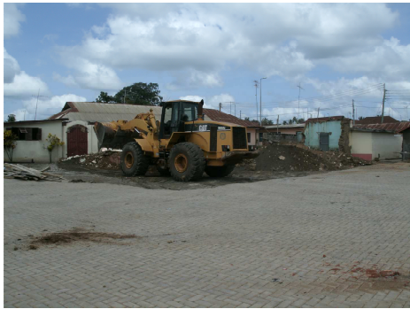
Fig. 4. A grader demolishing the old palace building, Ho-Bankoe (June 2012)
