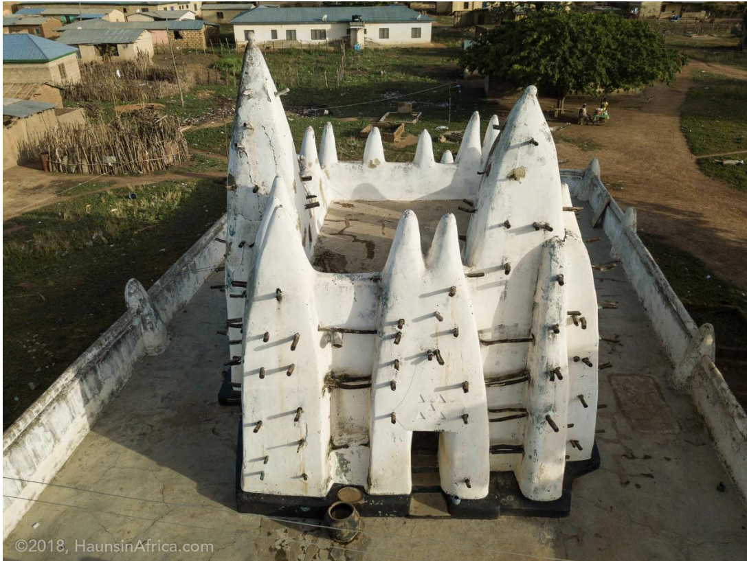
Figure 4.3-32: Aerial view of the front of Nakore Mosque. Source: HaunsinAfrica.com
