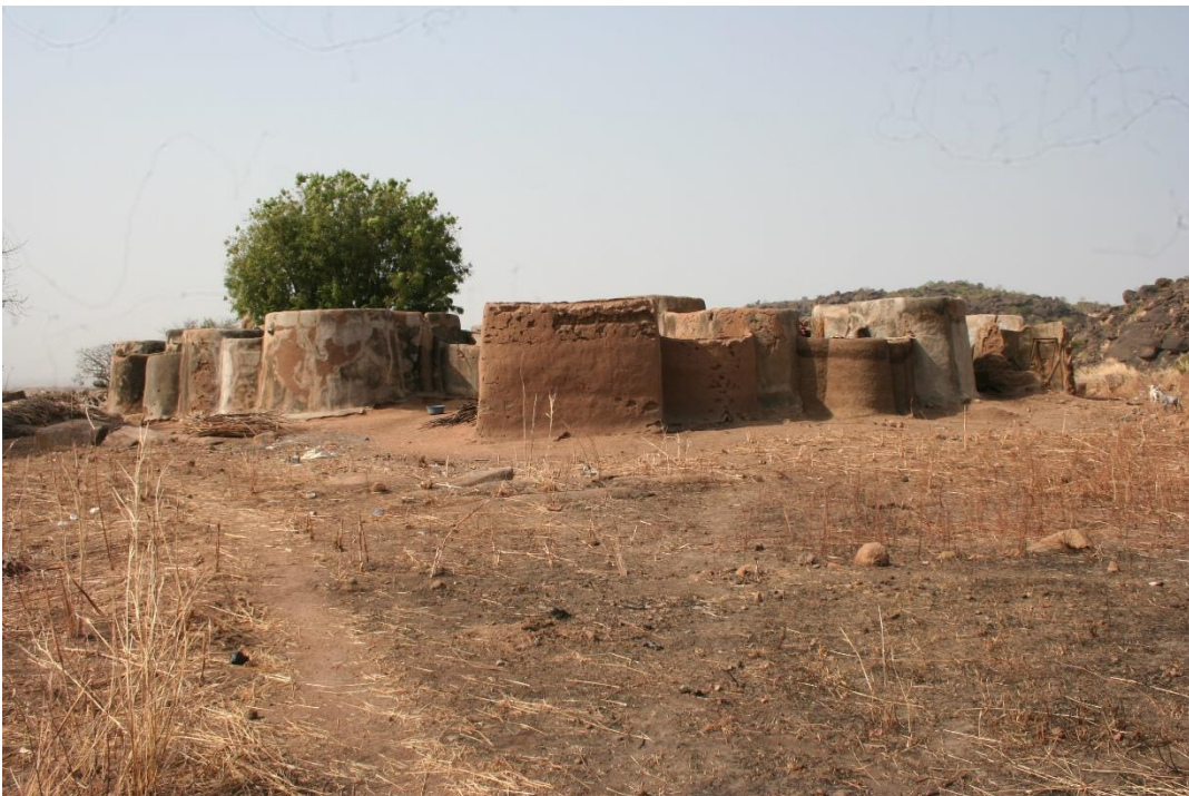
Figure 4.3-19: Tenzug architecture (Flat roofed). Source: Getrude Aba Mansah Eyifa Dzidzenyo
