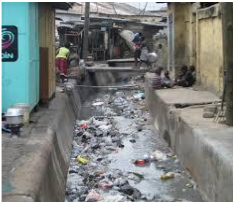
Plate 3: A section of the drainage system around the market
