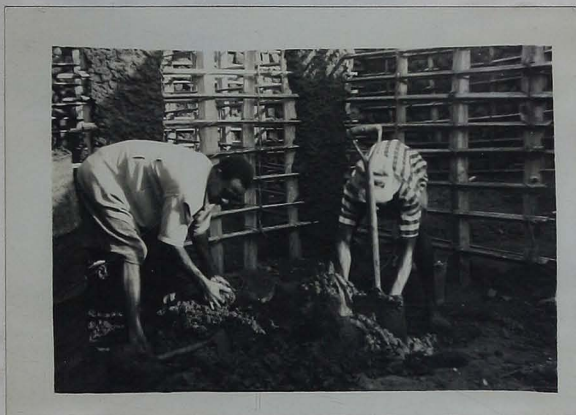
A swish building under construction
