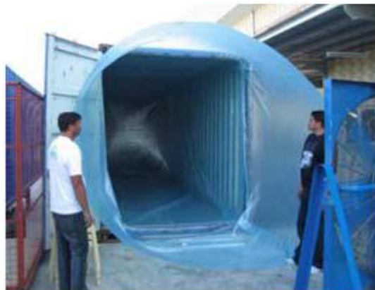
Plate 2. 3: TranSafeliner™ being installed in a shipping container
