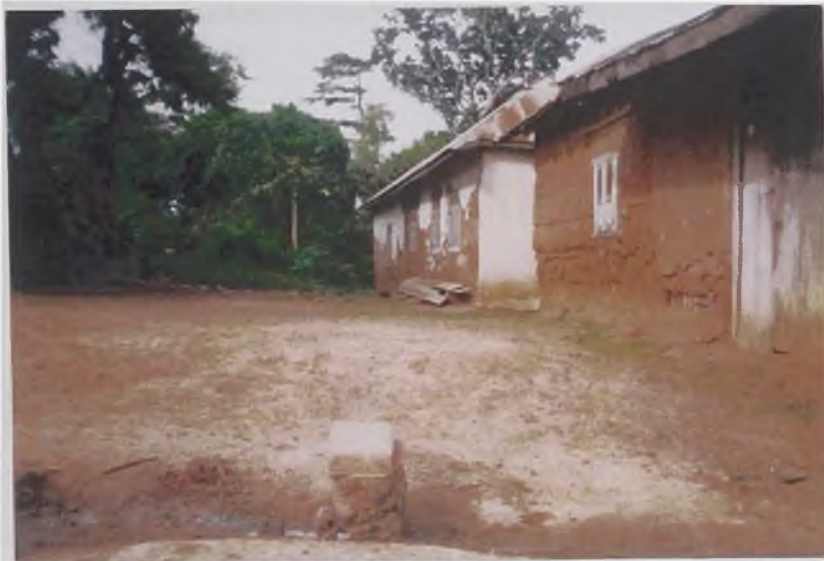
Plate 4.2: The location of a boundary pillar (in the foreground) lying several metres away from the present boundary at Kyeiase
