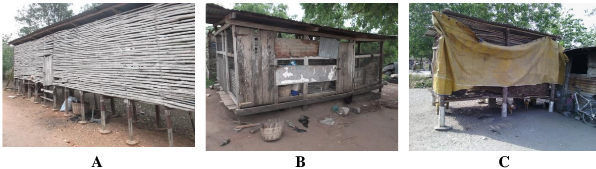
Plate 4.9 Crib Storage Structure made with (a) bamboo (b) sawn wood and wire mesh (c) with rodent-guards
