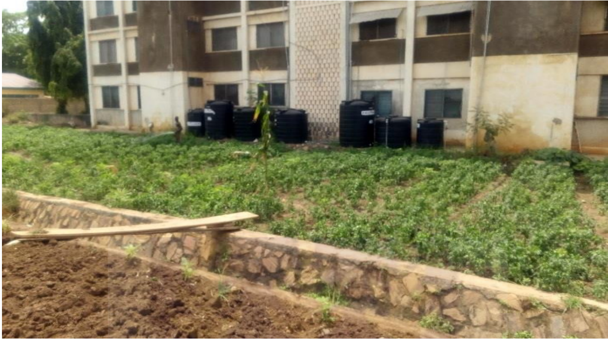
Plate 3.4 Open drain for sourcing waste water for irrigation.
