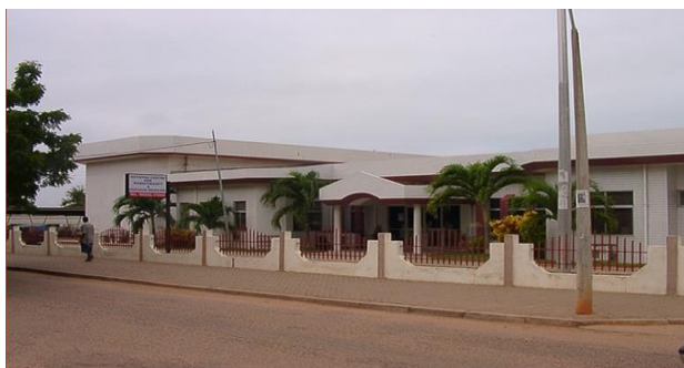
Fig. 3.1 The NCRONM building at KBTH
