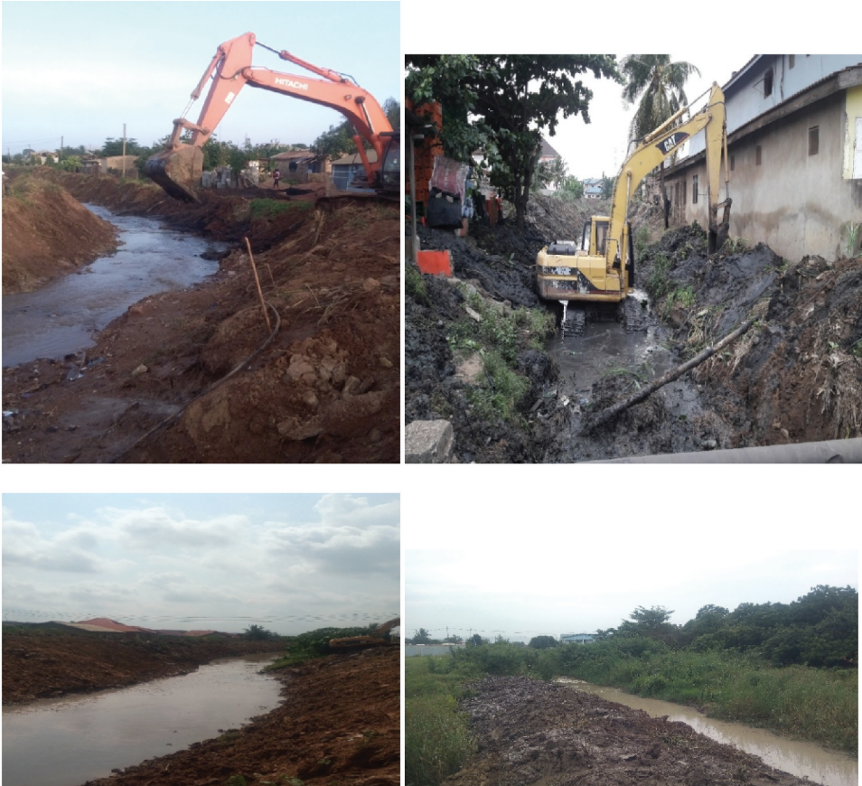
Figure 2. Samples of major dredging works in adentan municipal assembly. Source: NADMO Annual Report, 2020
