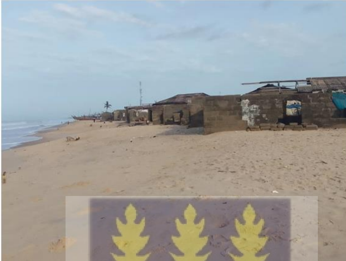
Picture depicting abandoned homes close to the coastline in the study area.
