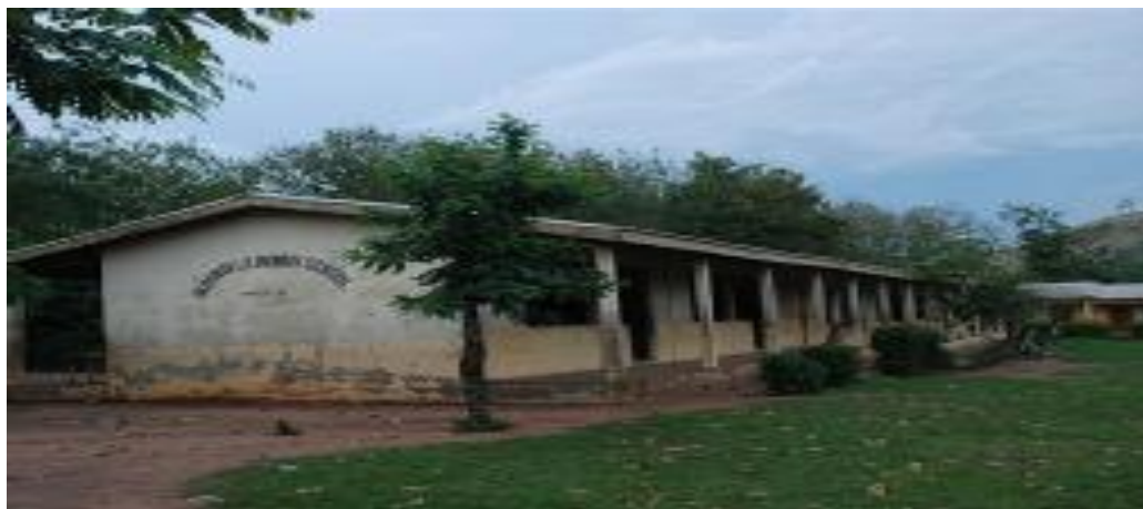
Plate 1: Picture of Akraman Primary School block before renovation
