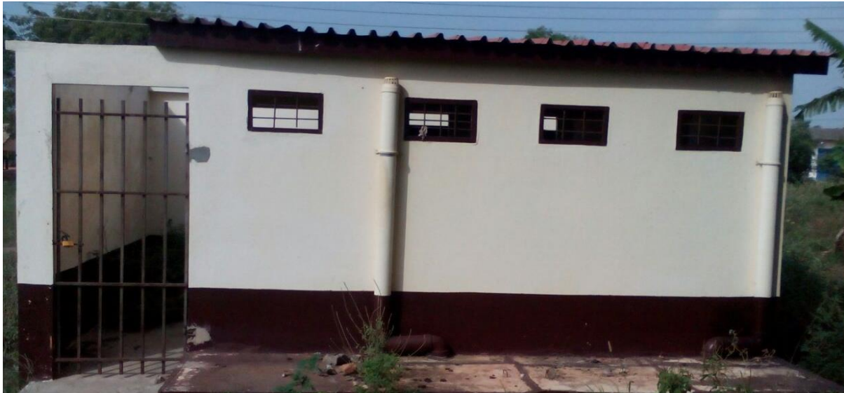
Plate 5: Toilet facility built for residents of Djankrom
