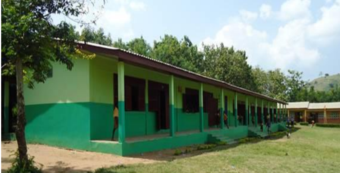
Plate 2: Picture of Akraman Primary School block after renovation
