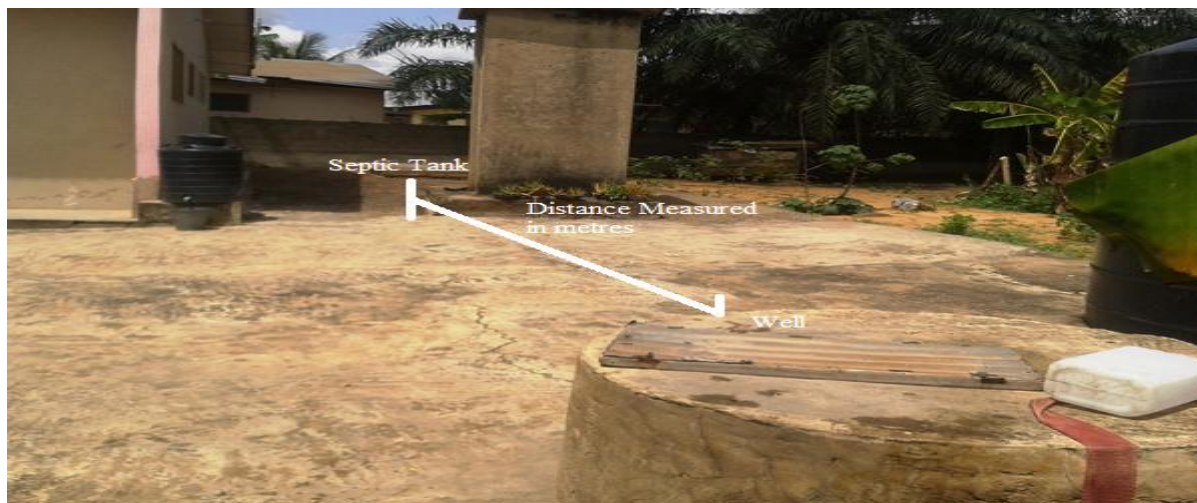
Plate 3. 1: Picture showing septic tank distance to well in a sampled residential household.
