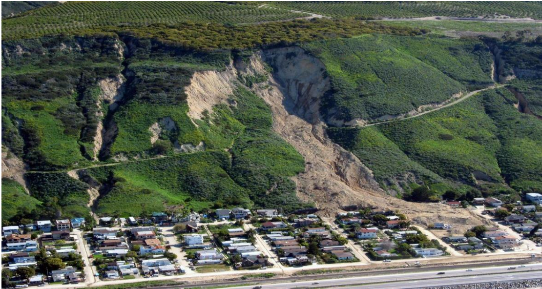
Plate 2.1: Mass wasting at La Conchita, California Source: USGS, 2016
