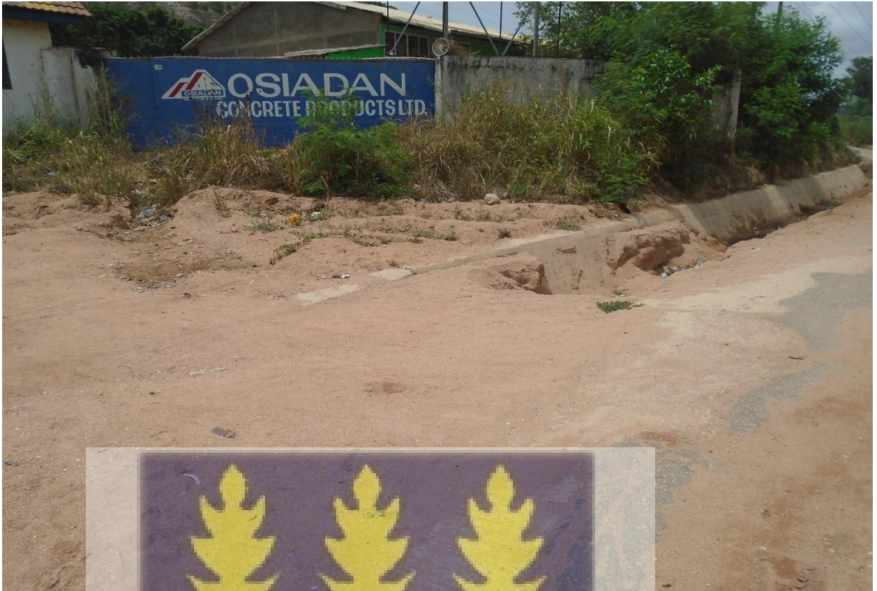
Plate 5. 8: Big Gutters Choked with Debris at around Osiadan Construction Limited Source: Author's Field Data, 2020
