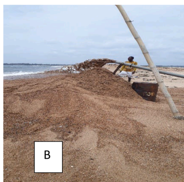
Sacks (40 feet long) filled with sand.
