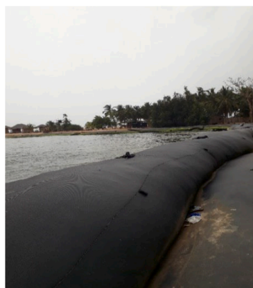
Sacks (40 feet long) filled with sand.
