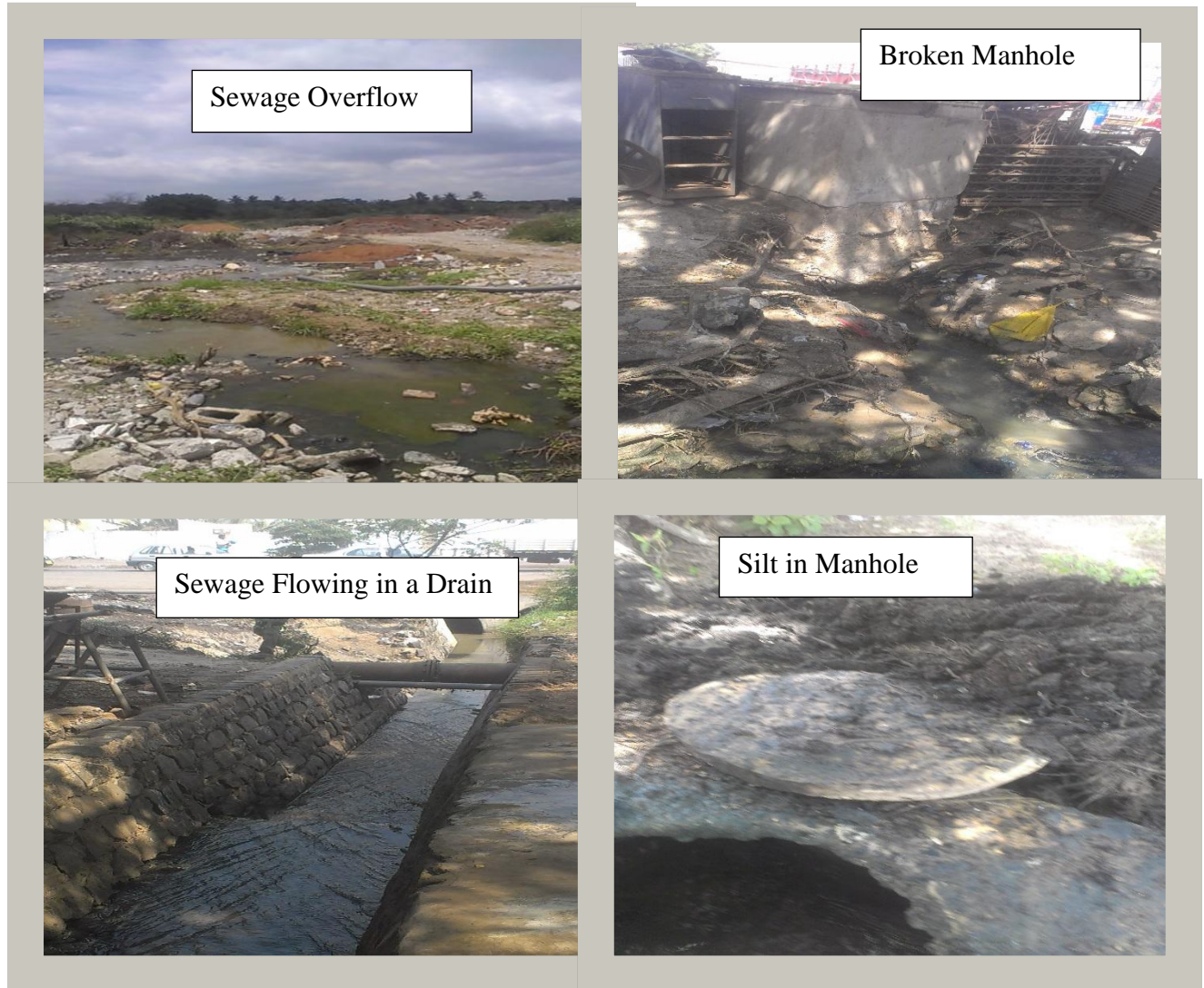
Plate 4.1 picture showing sewage pollution in the Tema Metropolis
