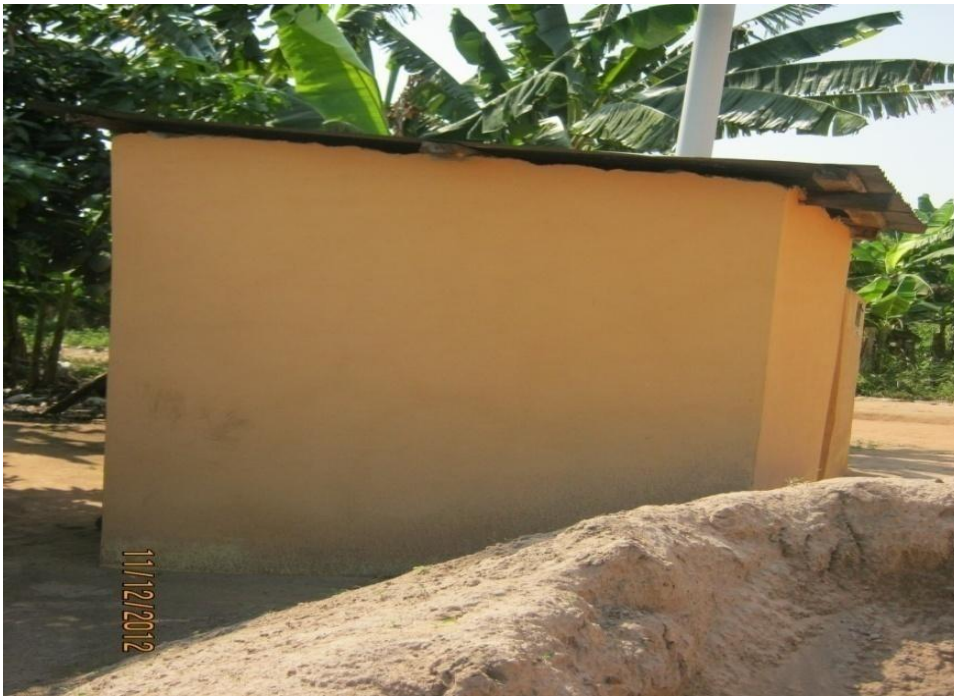
Picture 4: A Structure housing an NGO-financed KVIP
