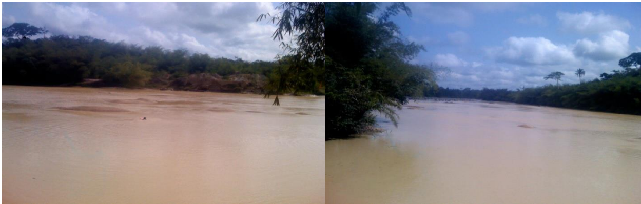
Plate 3.1: A section of the Lower Pra River at Daboase which is a current AGM site. Piles of sand located at the center of the river which aids in AGM operations.
