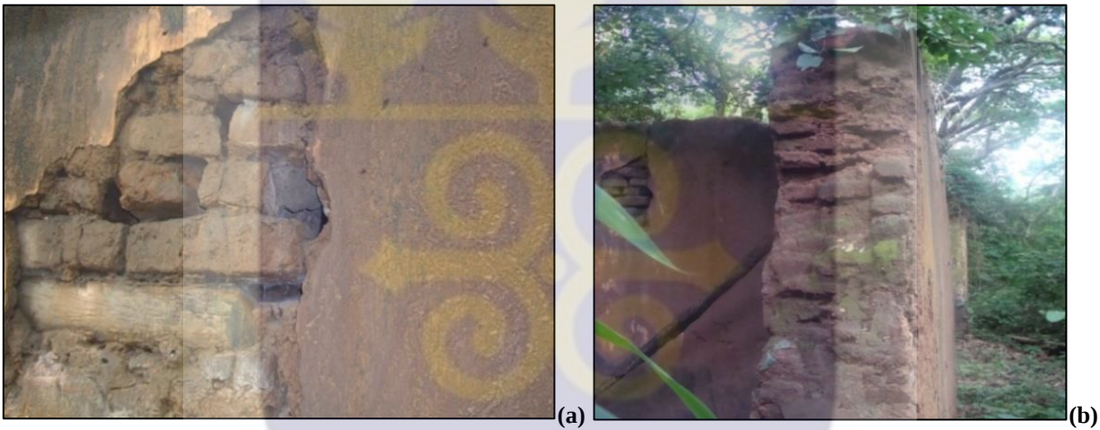
Figure 3.12 (a-b): Photo of the agor ti (Borassus trunk) in the locally made Bricks, as well as, the broken wall (Photo by Ms. Patricia Ayipey and Mr. Gideon Agyare).
