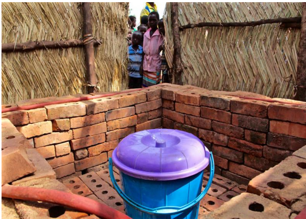
Figure 2.1: Structure of the ZECC
