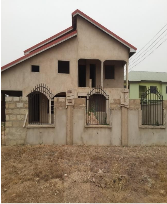
Plate 4.5: An uncompleted building in Community 25
