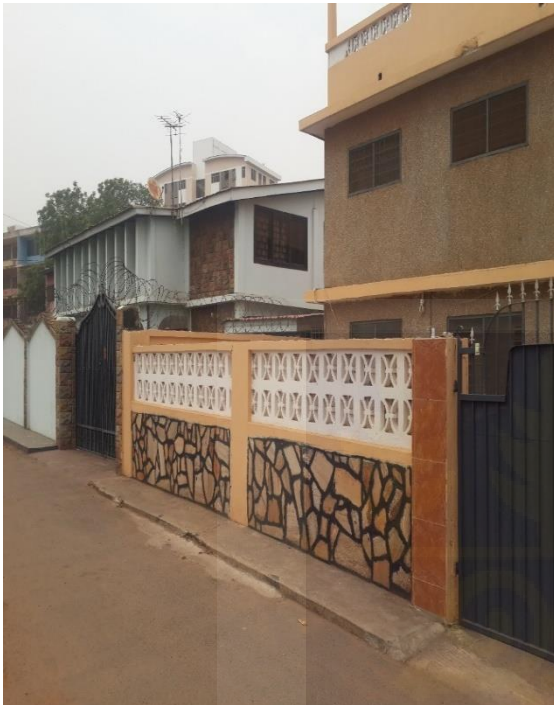
Plate 4.3: A typical altered TDC building at Community 1
